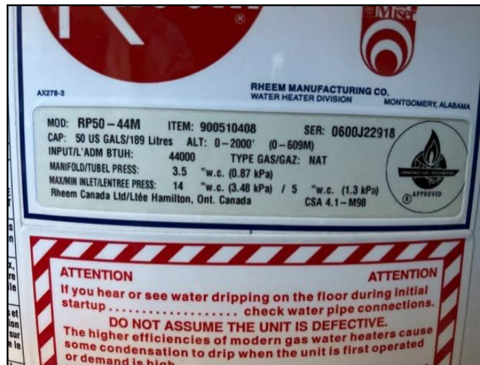
Water heater data plate
