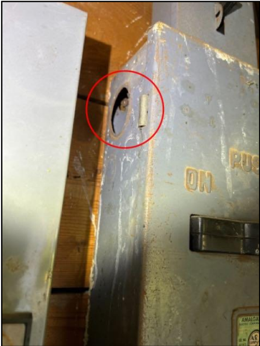
Unprotected openings
