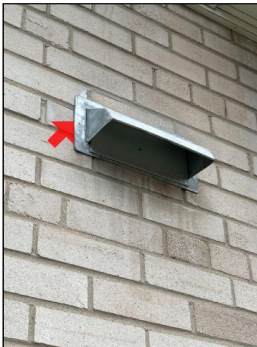
Caulking deteriorated/missing
