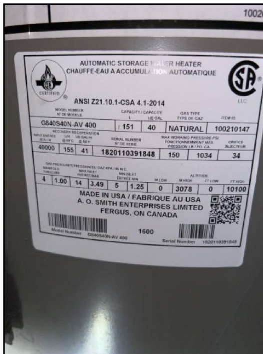
Water heater data plate
