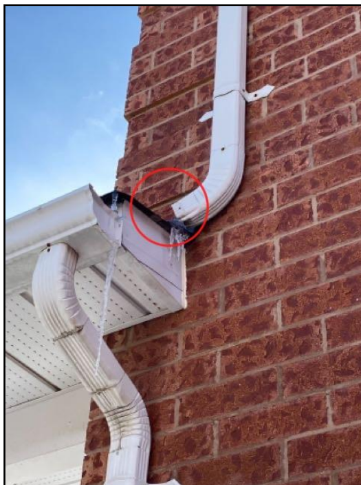
Discharge onto roofs
