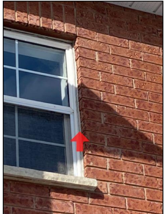
Caulking missing, loose or deteriorated
