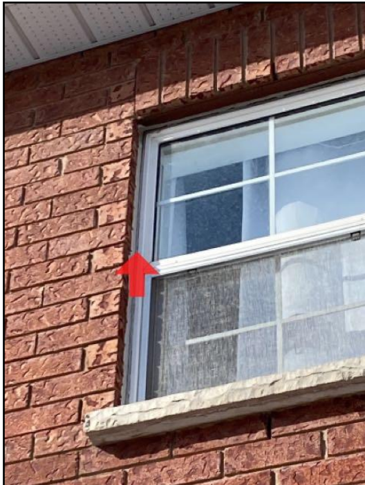
Caulking missing, loose or deteriorated
