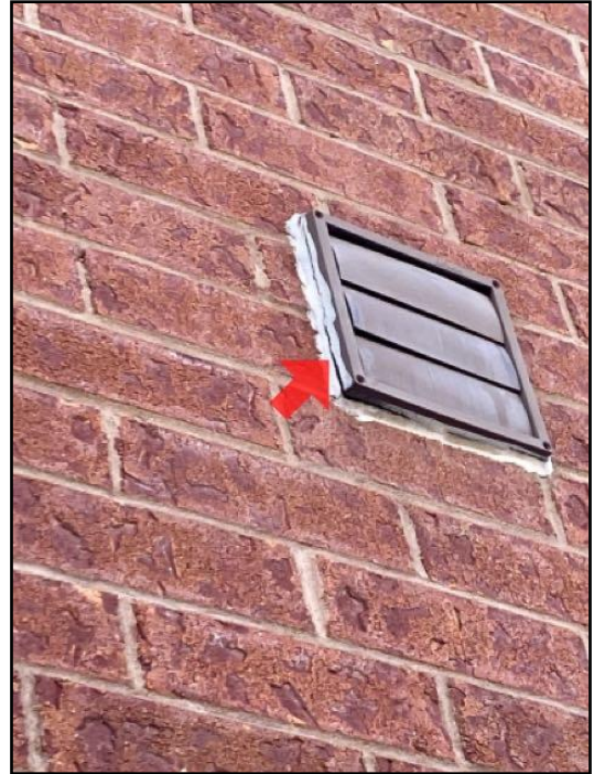
Caulking deteriorated/missing
