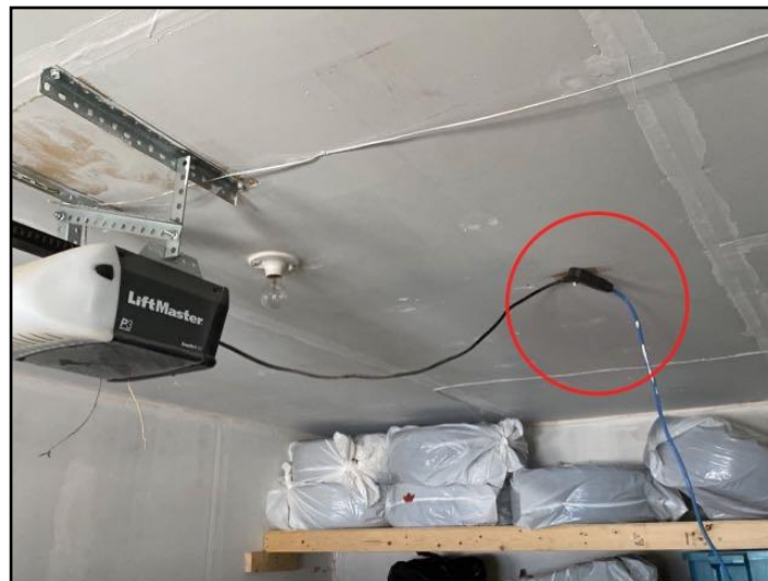
Extension cord for garage door operator...
