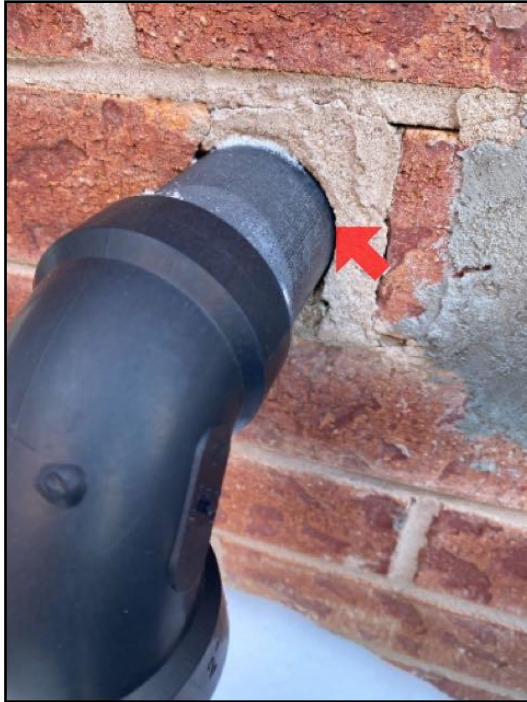
Caulking deteriorated/missing
