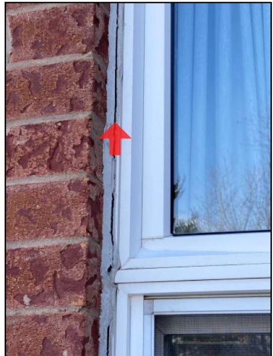
Caulking missing, loose or deteriorated
