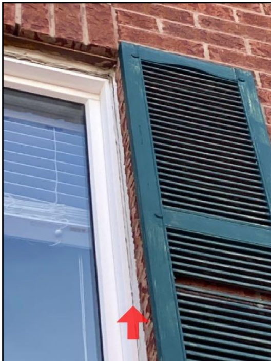
Caulking missing, loose or deteriorated
