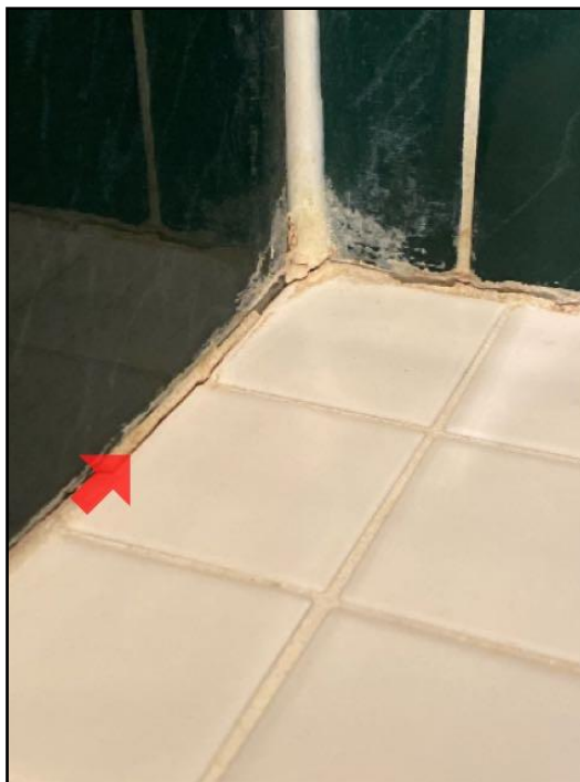
Caulking loose, missing or deteriorated
