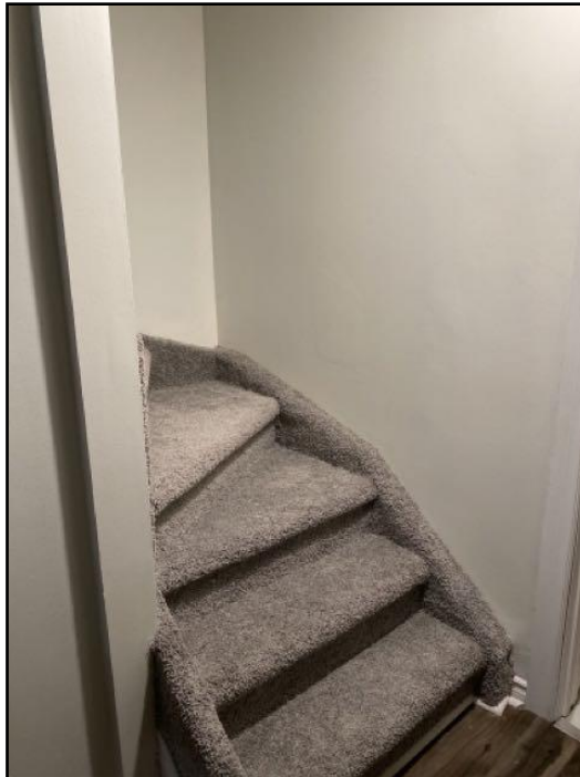
Missing handrail
