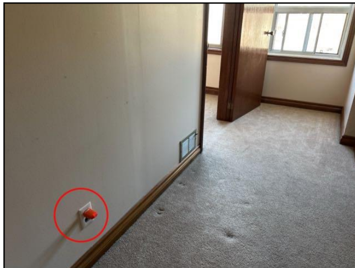
Reversed polarity
