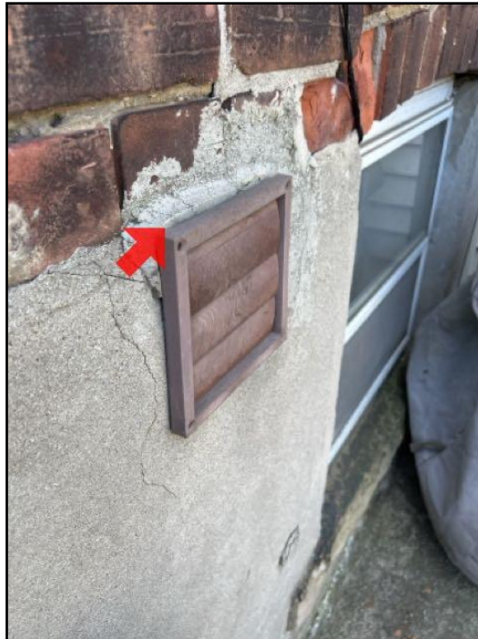
Caulking deteriorated/missing
