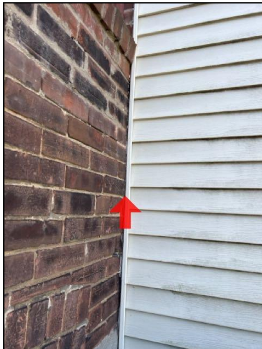
Caulking missing or ineffective
