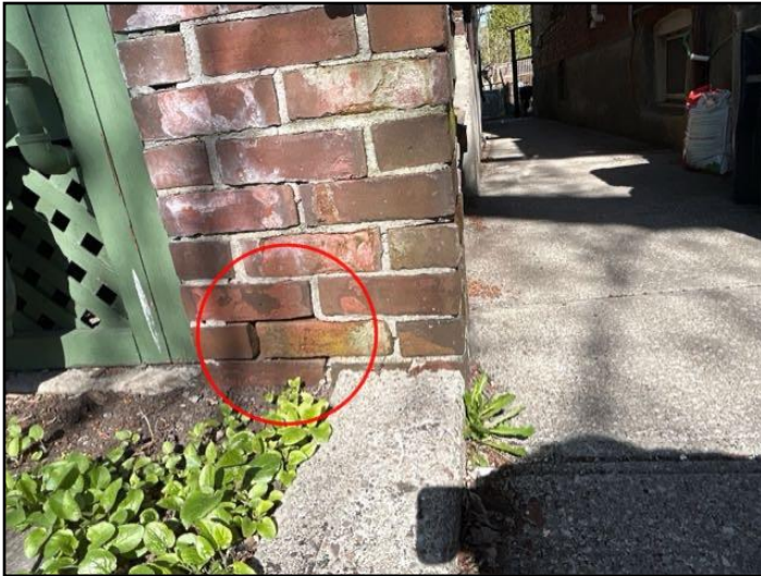
Mortar deterioration
