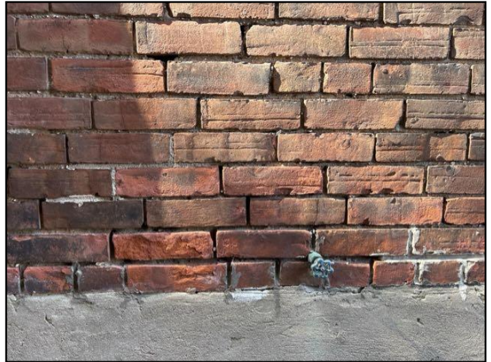
Mortar deterioration
