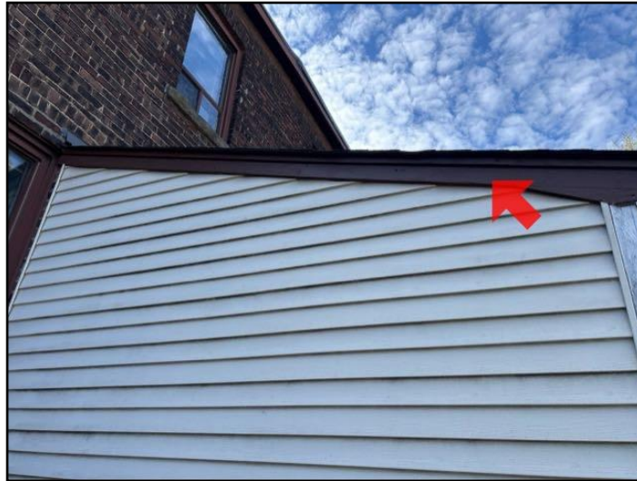
Flashings missing
