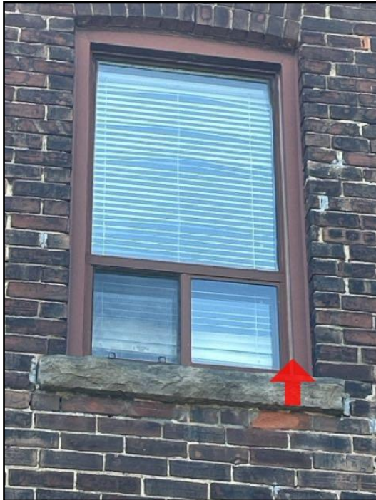
Caulking missing, loose or deteriorated
