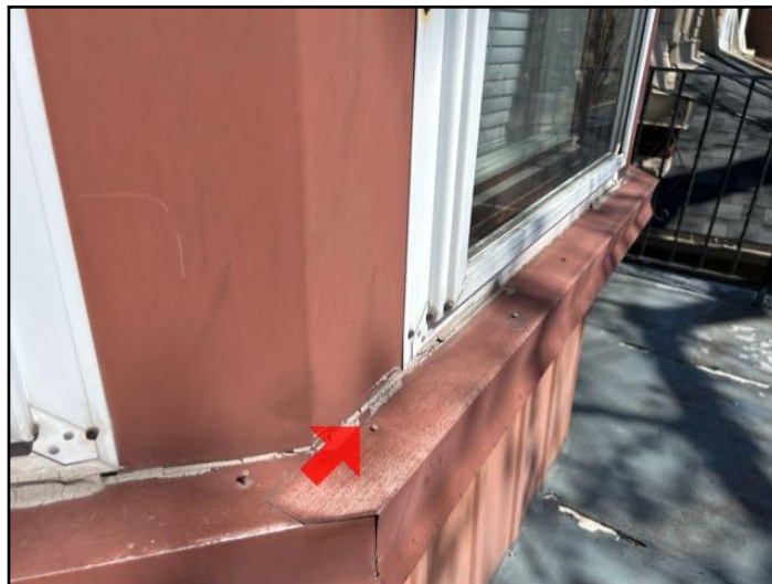
Caulking missing, loose or deteriorated
