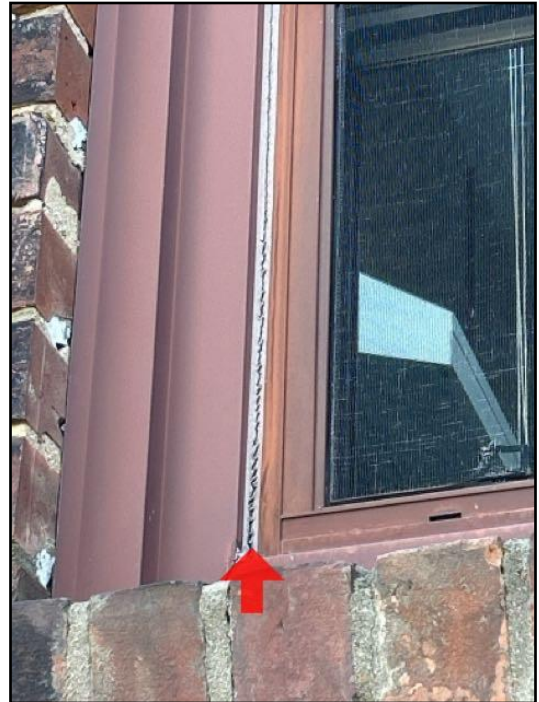
Caulking missing, loose or deteriorated
