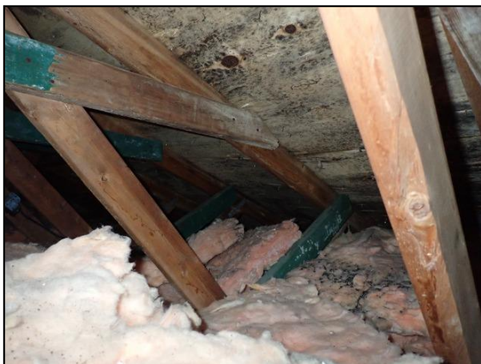
Mould on roof sheathing
