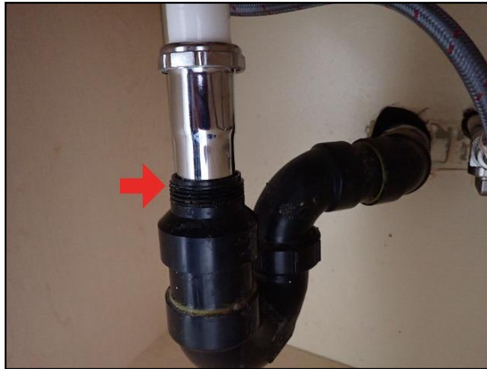
Tailpiece coupling nut missing
