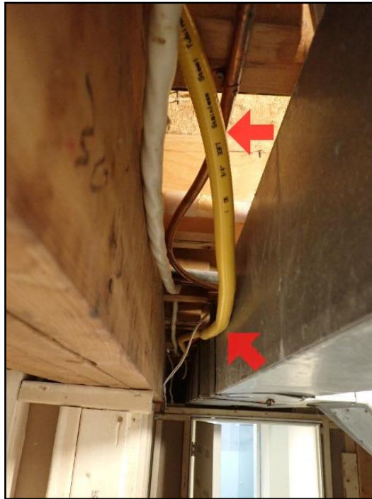
Loose support for gas line
