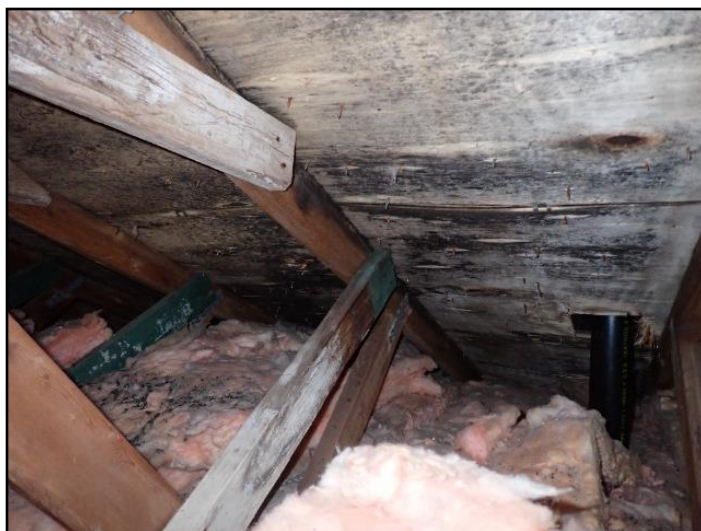
Mould on roof sheathing
