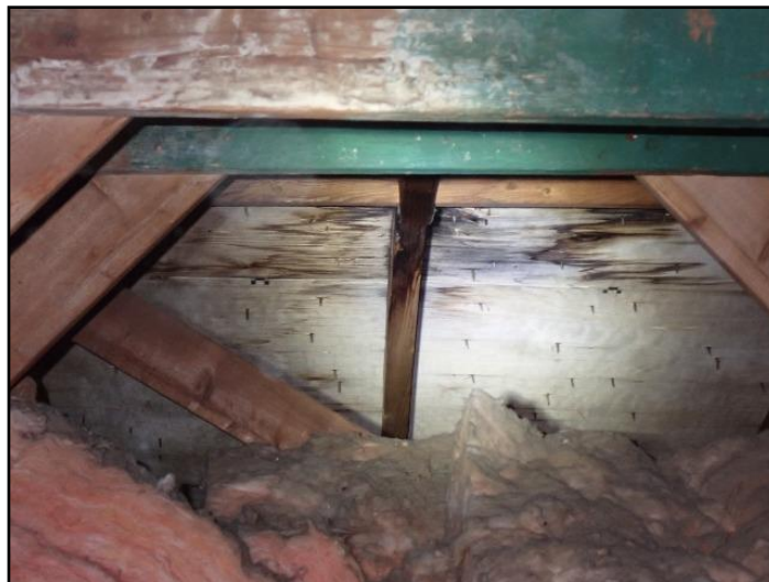
Water stains at the rear of the Attic
