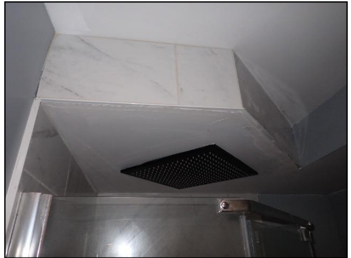
Rough finishing work on Bathroom ceiling
