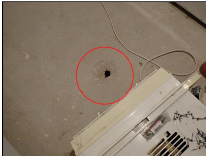
Obstructed floor drain
