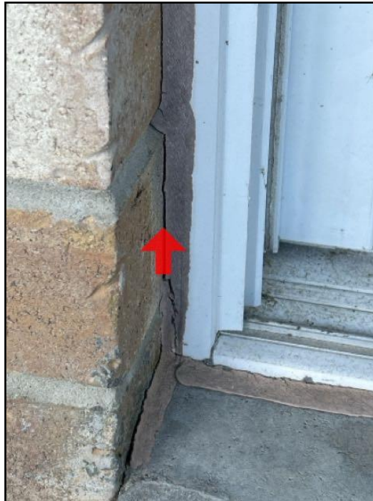
Caulking - deteriorated, loose or missing
