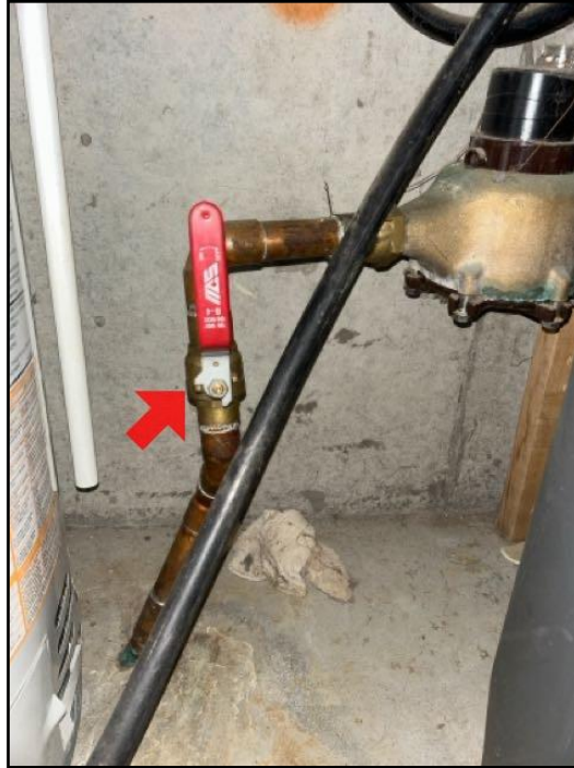
Water shut-off valve
