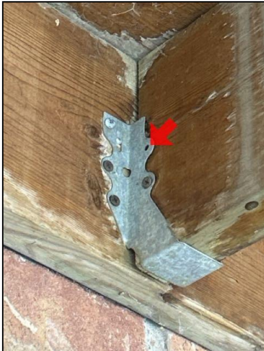
Missing fasteners
