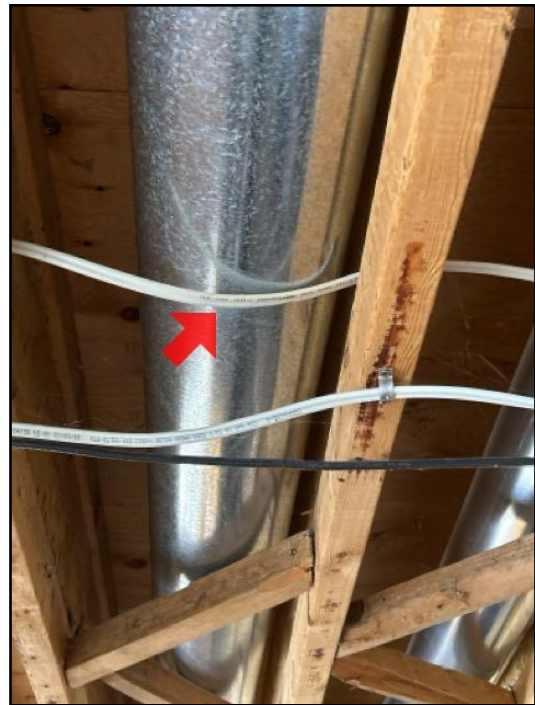
Too close to/touching duct, pipe, vent or...
