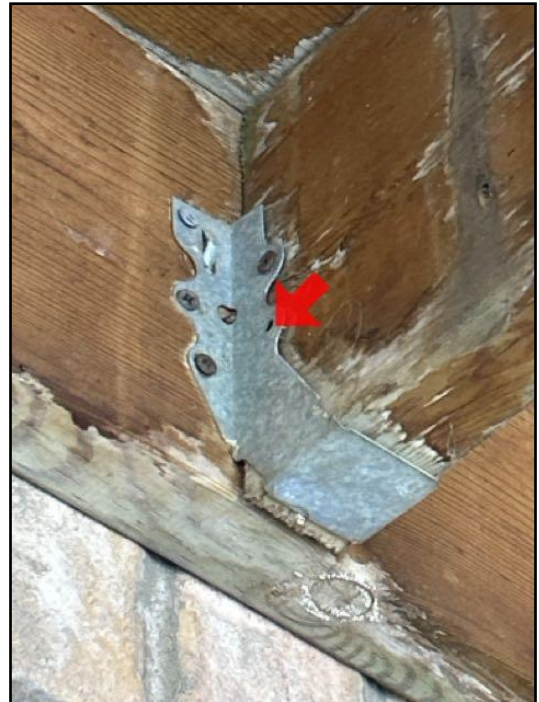
Missing fasteners
