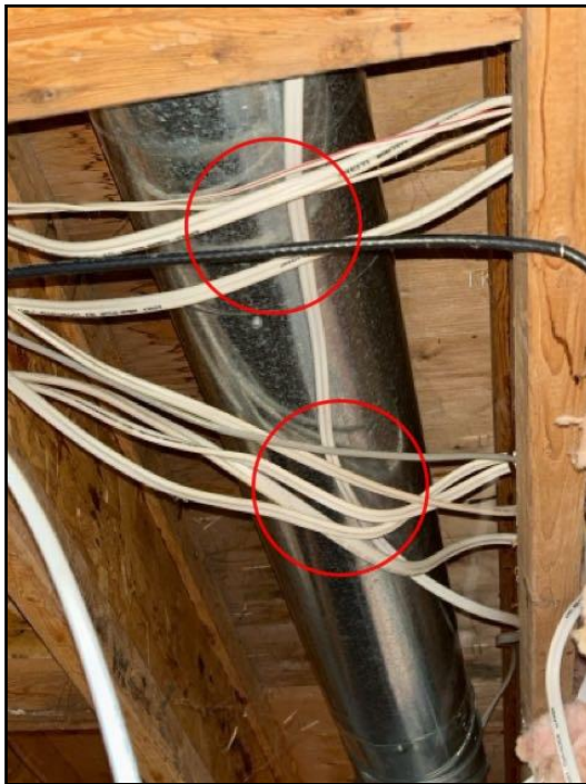
Too close to/touching duct, pipe, vent or...
