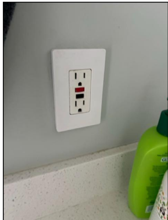
Test faulty on GFCI/GFI (Ground Fault...
