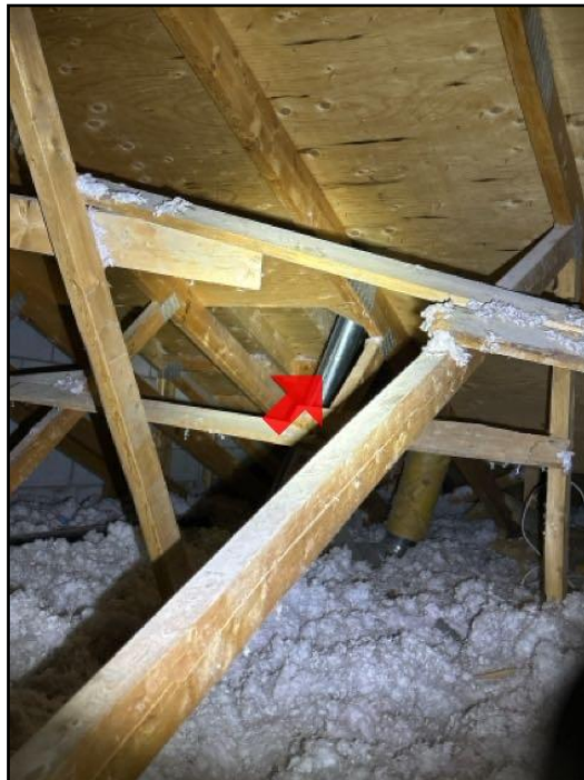
Not insulated in unconditioned space
