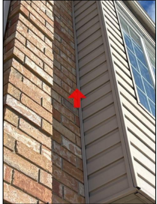
Caulking missing or ineffective
