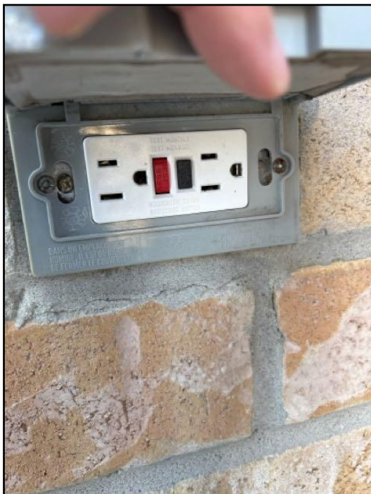
Test faulty on GFCI/GFI (Ground Fault...
