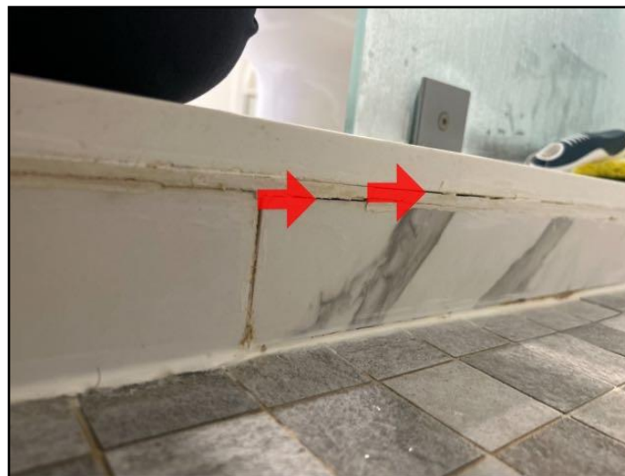
Grout loose, missing or deteriorated
