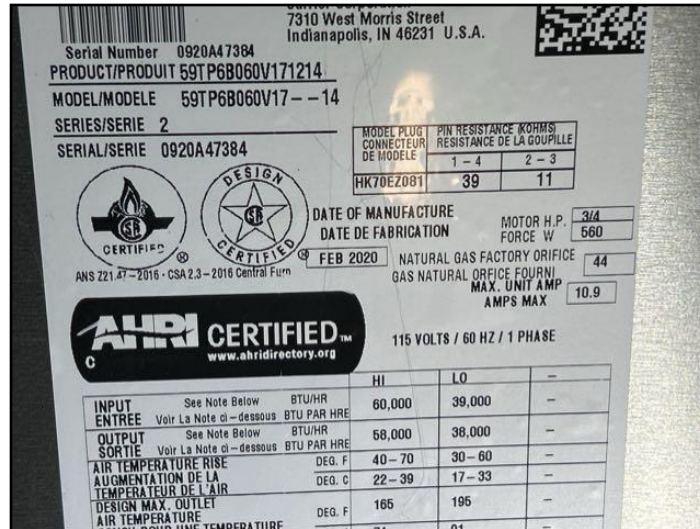
Furnace data plate
