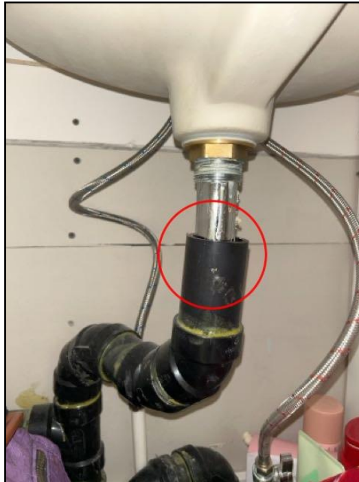
Drain assembly not properly installed
