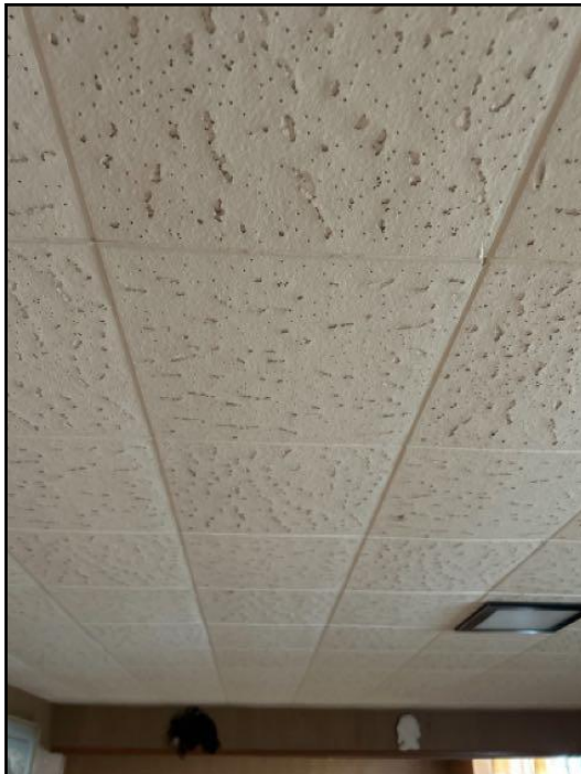
Possible asbestos containing materials
