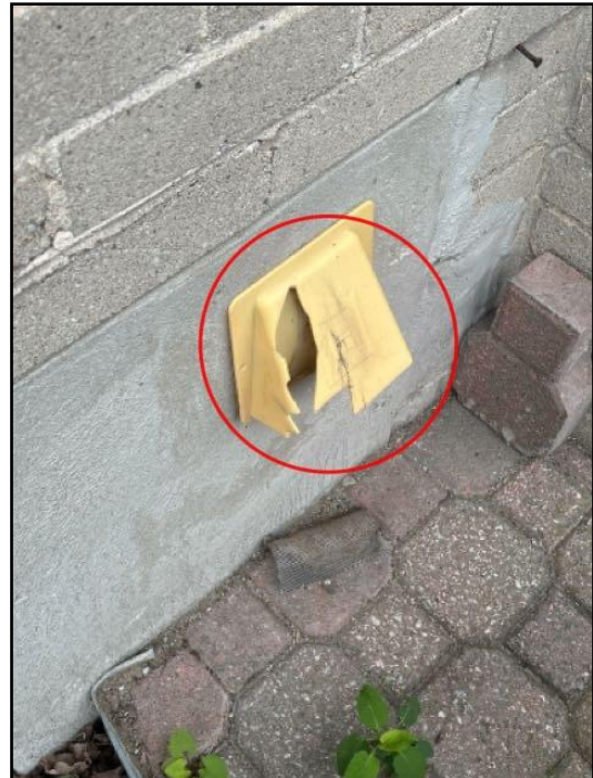
Cover damaged
