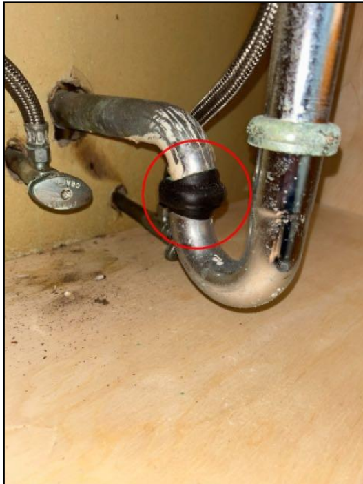
Possible poor seal/leak
