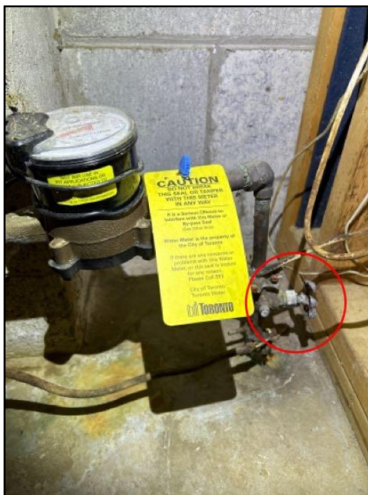
Water shut-off valve
