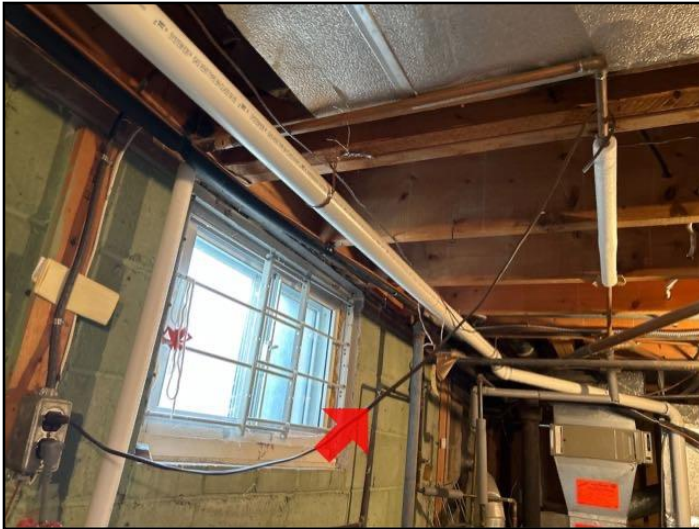
Extension cord used as permanent wiring
