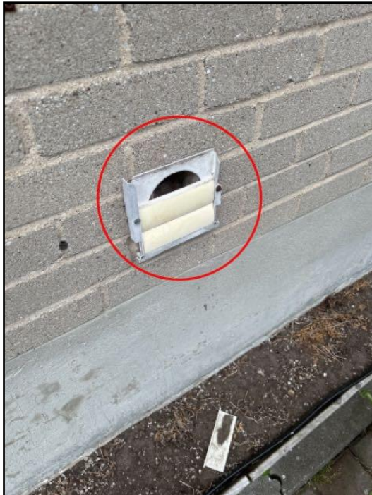
Cover damaged
