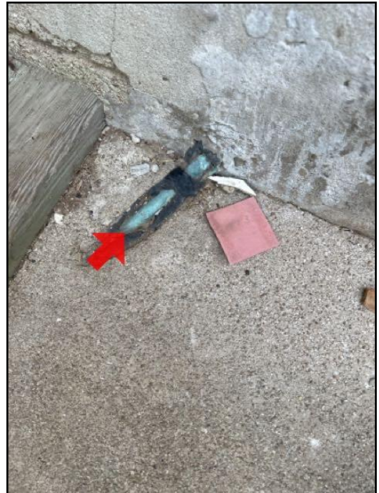
Insulation damaged/missing
