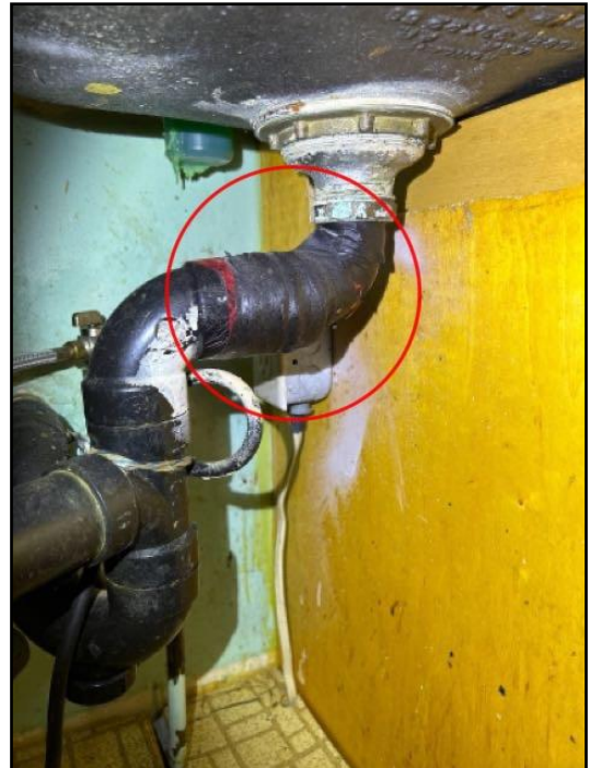
Possible poor seal/leak
