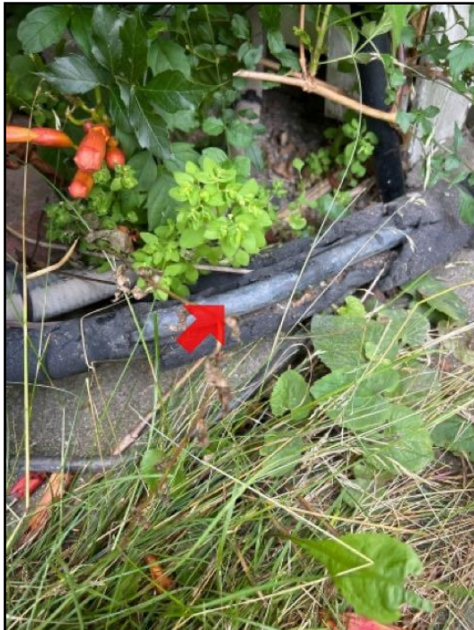
Insulation damaged/missing
