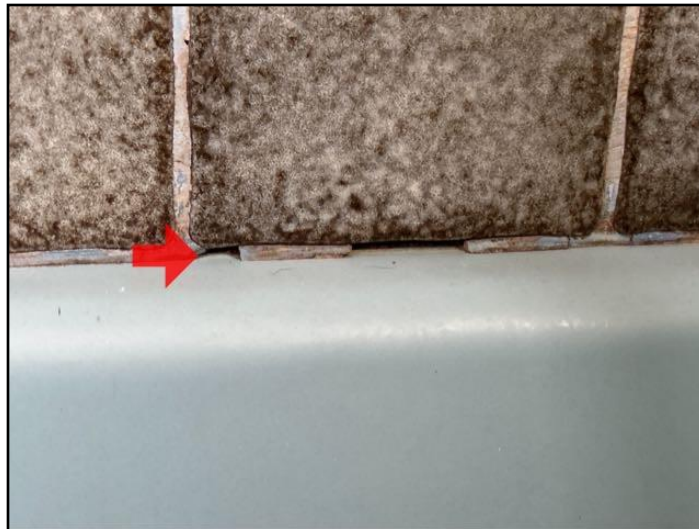
Caulking loose, missing or deteriorated
