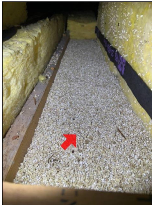
Vermiculite insulation
