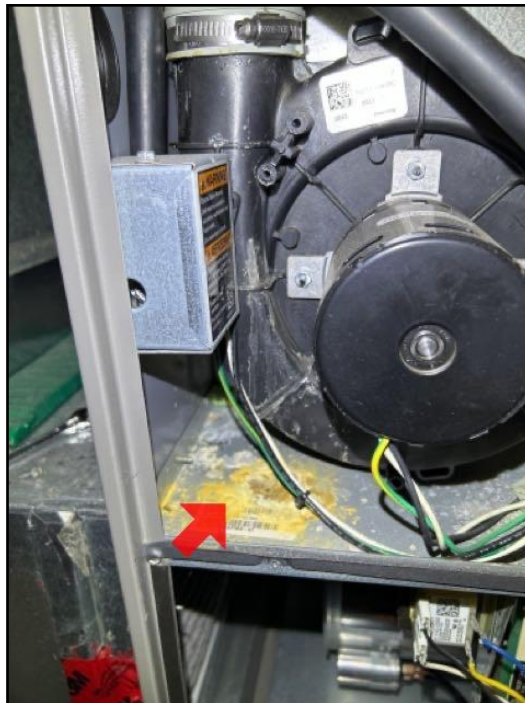
Condensate leak
