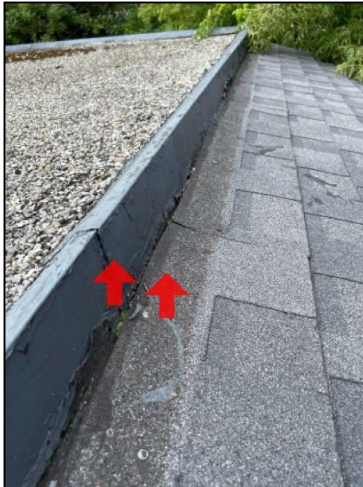
Missing flashing
