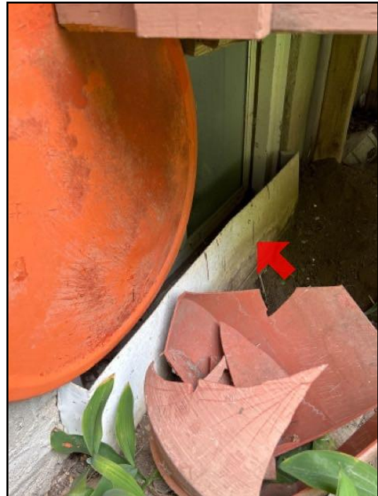
Missing/inadequate window well
