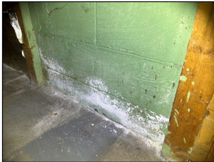
Efflorescence
