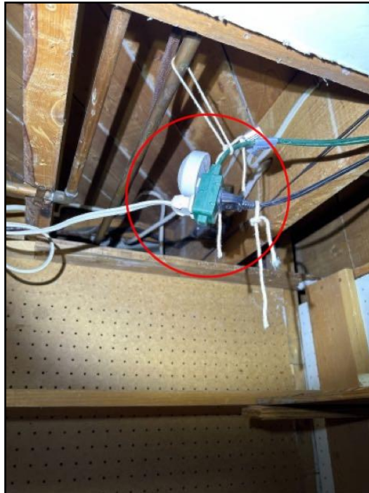
Extension cord used as permanent wiring
