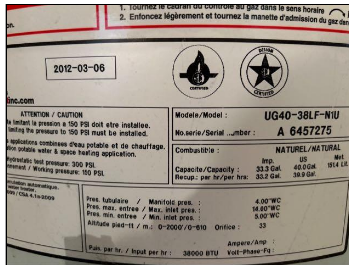
Water heater data plate
