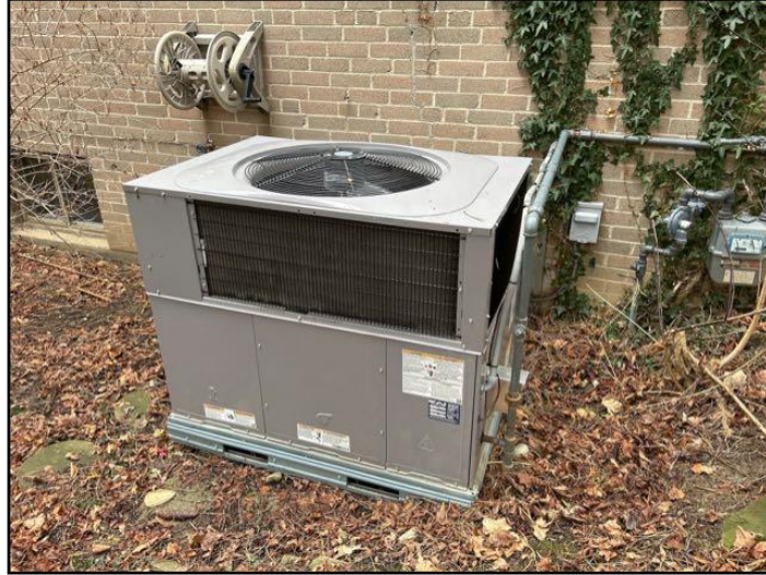
Integrated furnace and air conditioner
