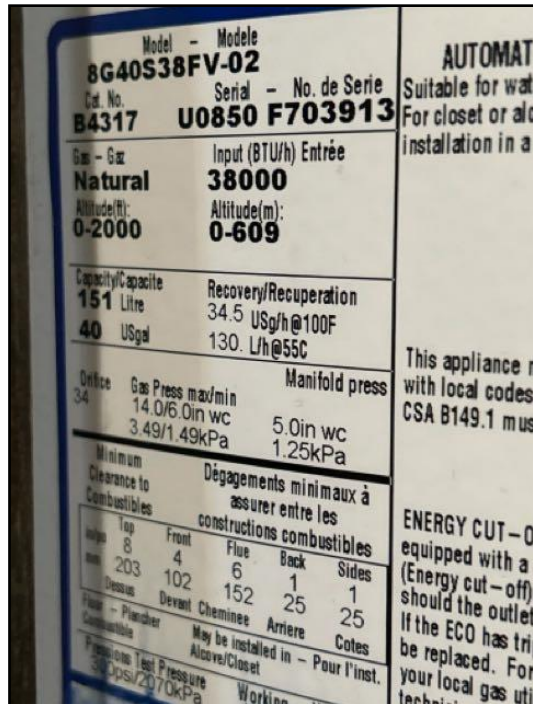
Water heater data plate
