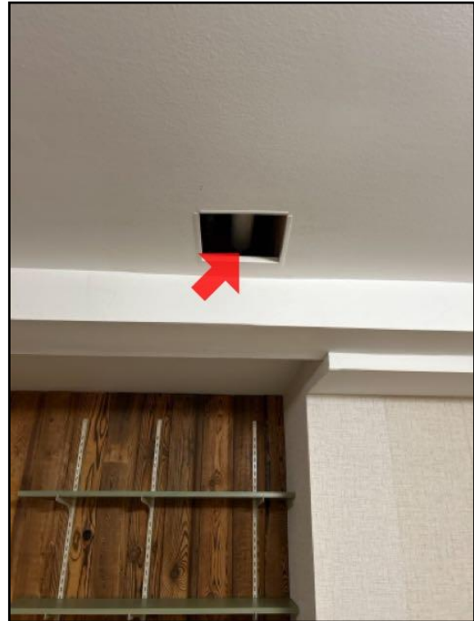
Water shut-off valve
