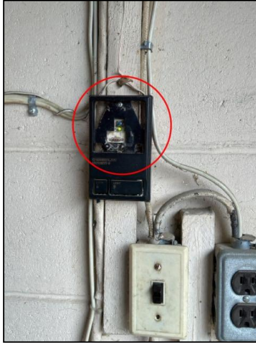
Switch damaged
