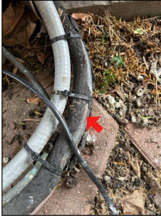
Insulation damaged/missing
